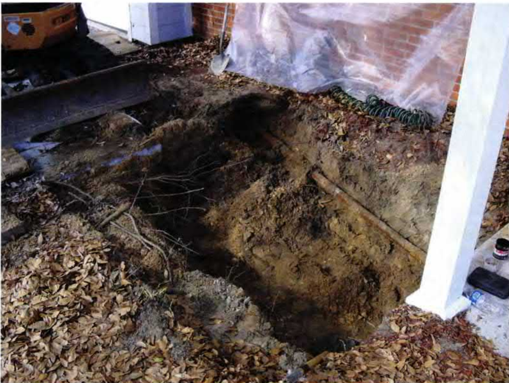
Picture 2: UST 1349Cardinal excavation in progress.
